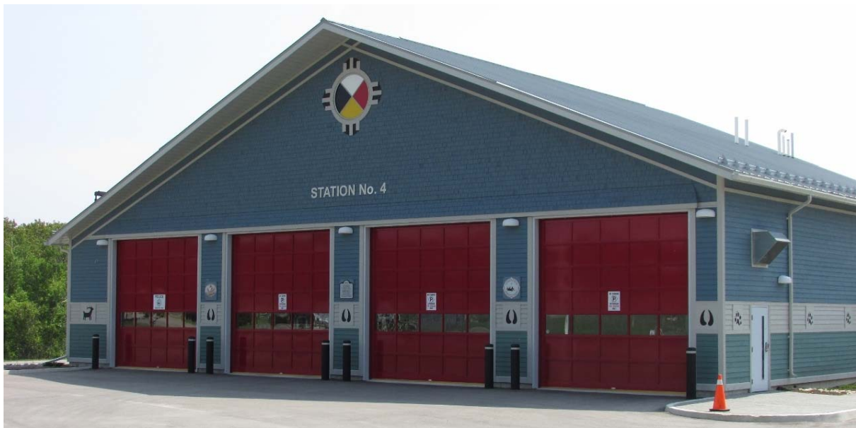
PHOTO TAKEN OF THE TRUCK BAY BUILDING ELEVATION.
