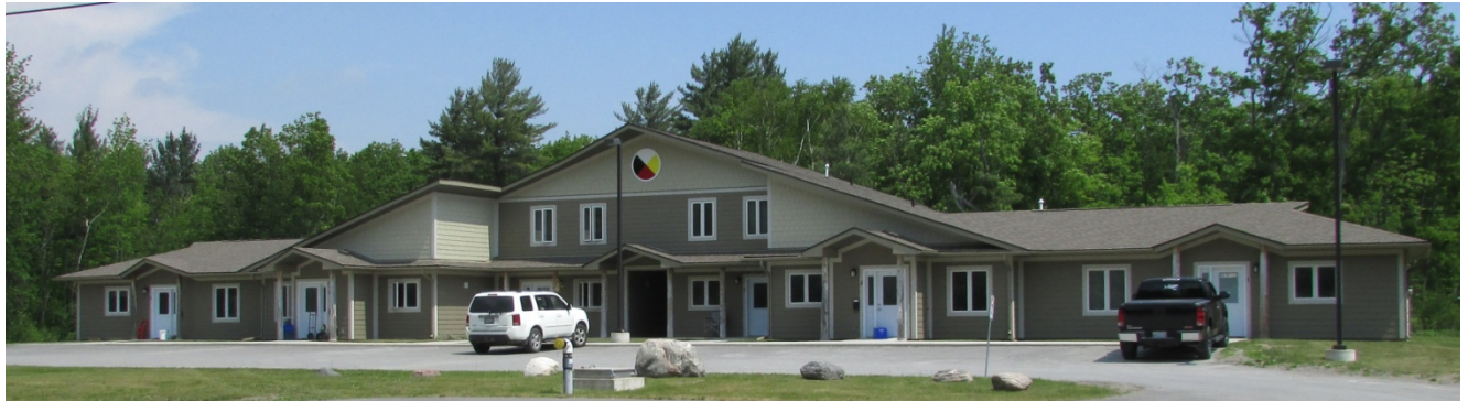
PHOTO TAKEN OF THE SOPER'S LANE BUILDING ELEVATION.
